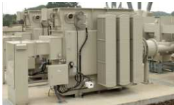
Eco-friendly palm fatty acid ester-immersed transformer
