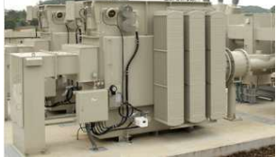
Eco-friendly palm fatty acid ester-immersed transformer
