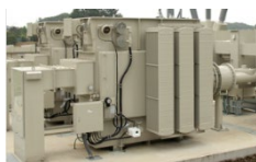
Eco-friendly palm fatty acid ester-immersed transformer
