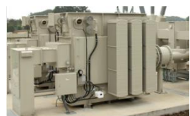
Eco-friendly palm fatty acid ester-immersed transformer
