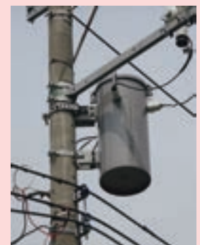
Pole-mounted transformer
