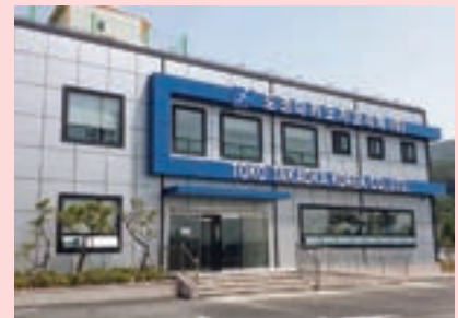
Exterior view of the plant at TAKAOKA TOKO KOREA CO., LTD.
