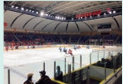
The completed Hakucho Oji Ice Arena We installed LED lighting in the ceiling and the electronic scoreboard on the far right.
