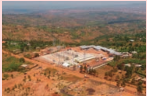
The completed Gasogi substation
