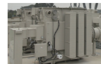
72 kV transformer
