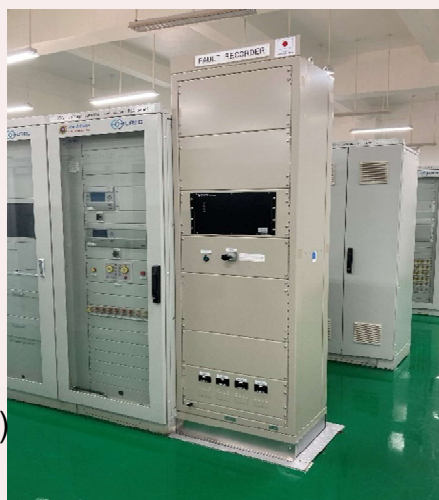
Oscillograph data recording device (Dongphosy substation)
