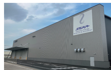
Meter Equipment Center exterior
