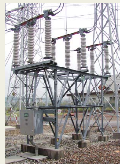
Horizontal double break disconnecter (THR5/6)
