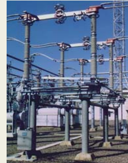
300kV Horizontal center break disconnecter
