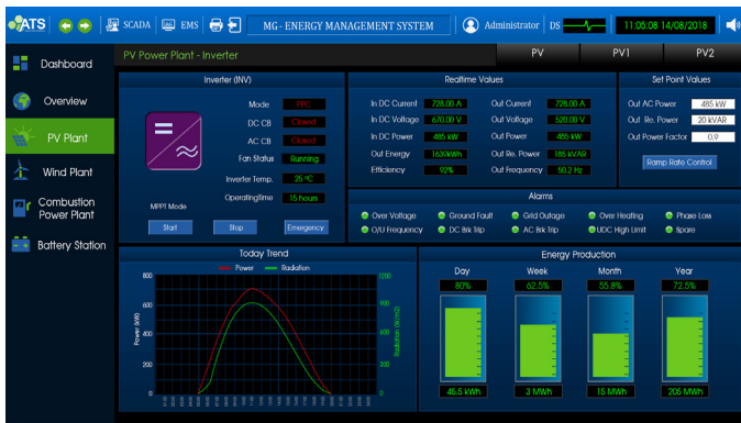
Figure 21. Specific Inverter unit
