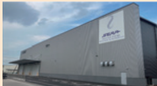
(Figure 1) Exterior of the Smart meter assembly & delivery center
